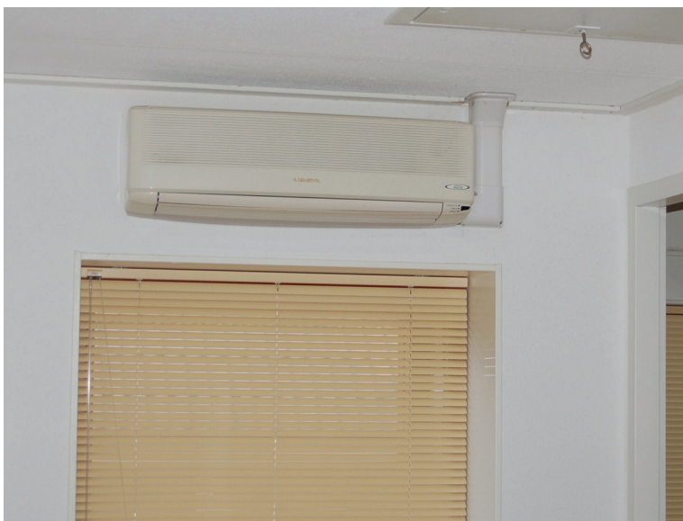
Afb. C.2 Binnenunit split-unit wandmodel
