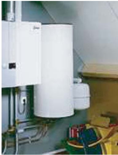
Afb. 3.36 Boiler indirect gestookt
